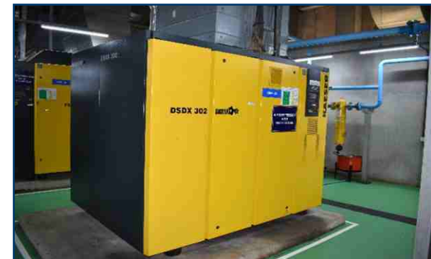
Air Cooled Screw Compressors
