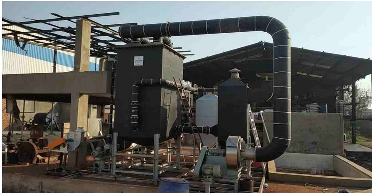
TRL-RAIN™ Installed on Site
