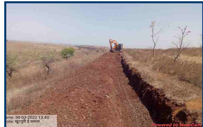
Development of water absorption trench in Khutpuri village, dt. Buldhana, Maharashtra
