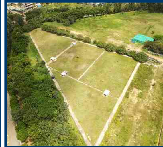
Underground Tank-3 33,000 KL Capacity
