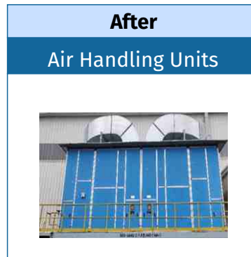
Air Handling Units does not require water for shop floor cooling
