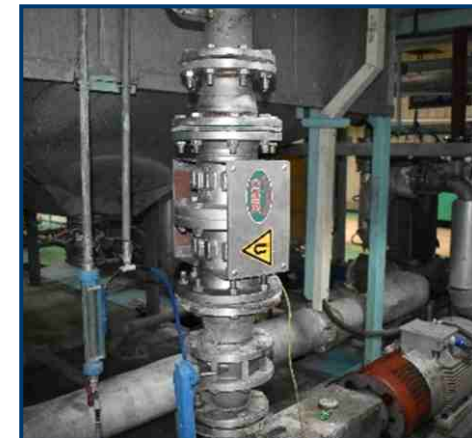
Magnetic Module Installation
