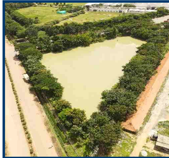
Open Water Tank-2 23,000 KL Capacity
