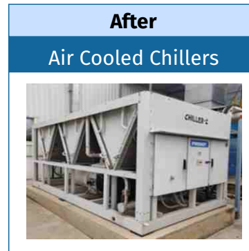
Air Cooled Chillers does not consume water
