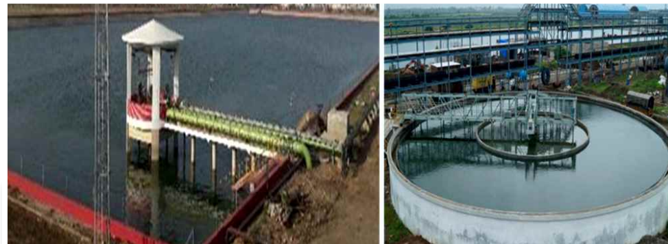
Rain water harvesting and reuse in process
