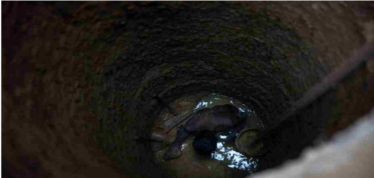
Well digger digging a well
