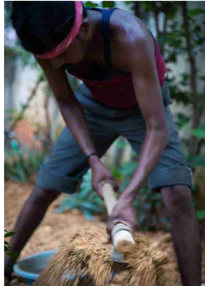
Well digger digging a well
