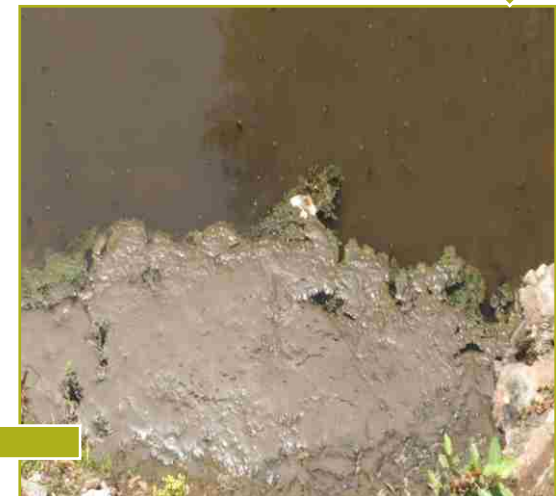
Bio-dredging in progress
