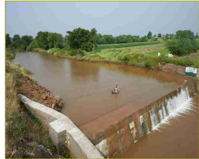
Check Dam - Pune dt., Maharashtra
