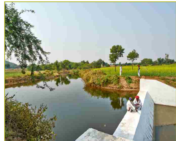
Check dam Pratapgarh dt. Rajasthan
