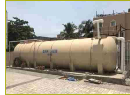
Commercial Building (40KLD)
