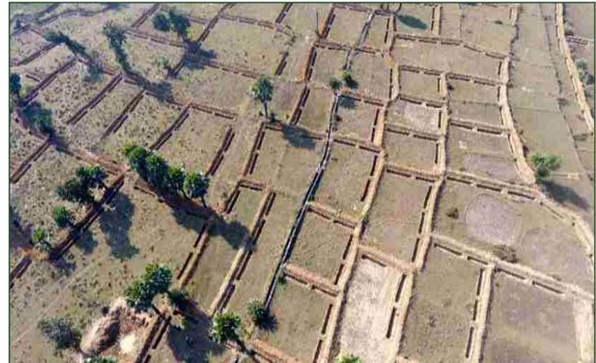
Trench cum Bund (TCB) Constructed in Village – Barmuri of Keliasole Block at Dhanbad District of Jharkhand State.
