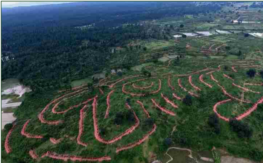
Water Absorption Trench (WAT) Constructed in Village – Parasi of Ichak Block at Hazaribagh District of Jharkhand State
